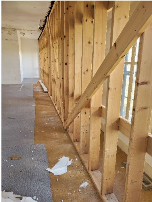
Figure 9. Cameron House Interior (Temporary support installed to stabilize the structure)
