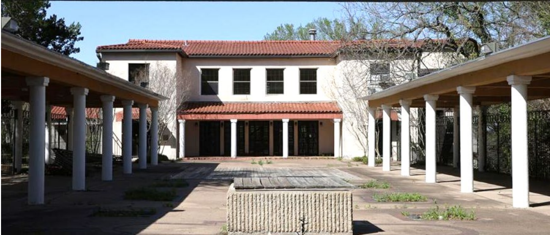
Figure 6. Cameron House Courtyard (South Side)
