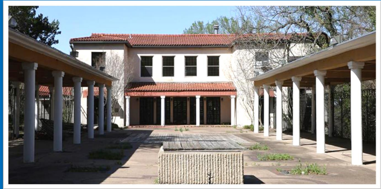
Cameron House (South Side)
